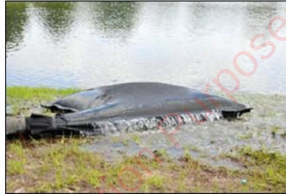
Plate 2-2 Silt bag under inspection
